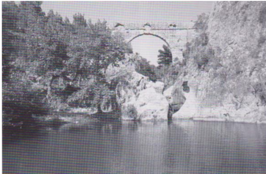
Figure 4. The big bridge in the Kemerdere valley (Aylward et al., 2002)
