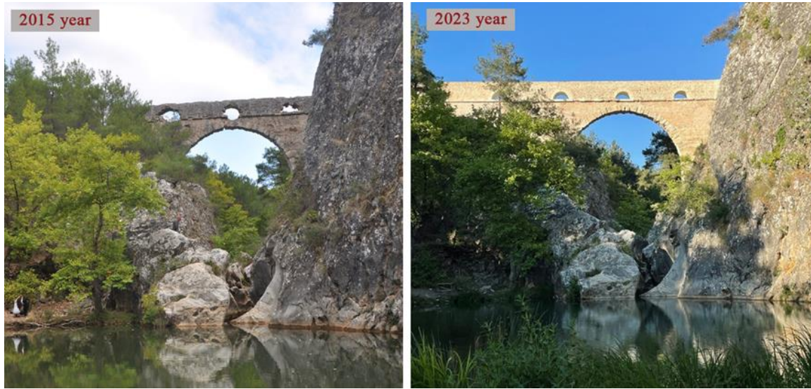
Figure 10. Images of the Kemerdere Aqueduct before and after restoration (Original, 2023)
